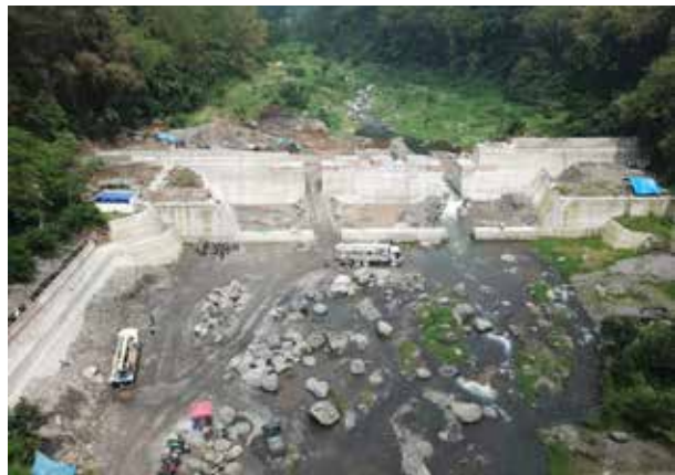
Sabo Dam Merapi
