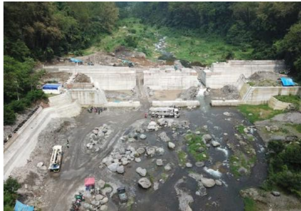
Sabo Dam Merapi
